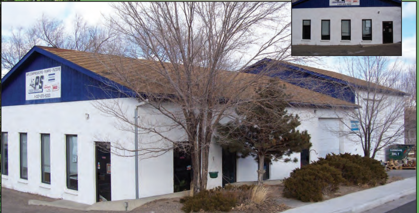
Power Service of Green River Store
